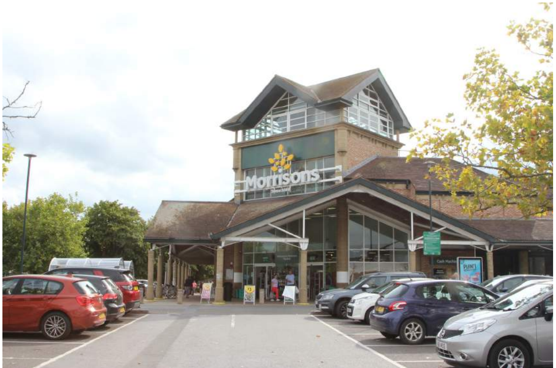
Figure 4.7: Photograph of Morrisons and Priory Bridge Road TCA
